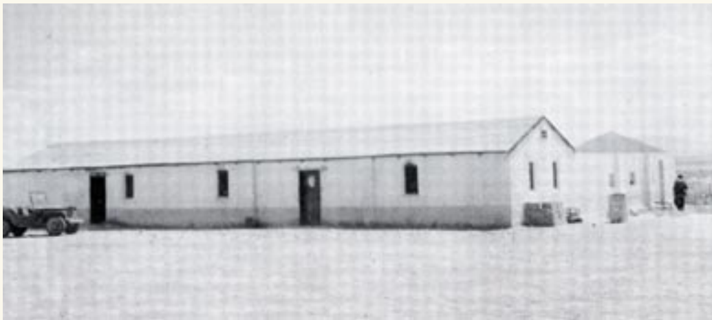
This building housed both the Orderly Room and the Enlisted Club of the 73 rd BS.
