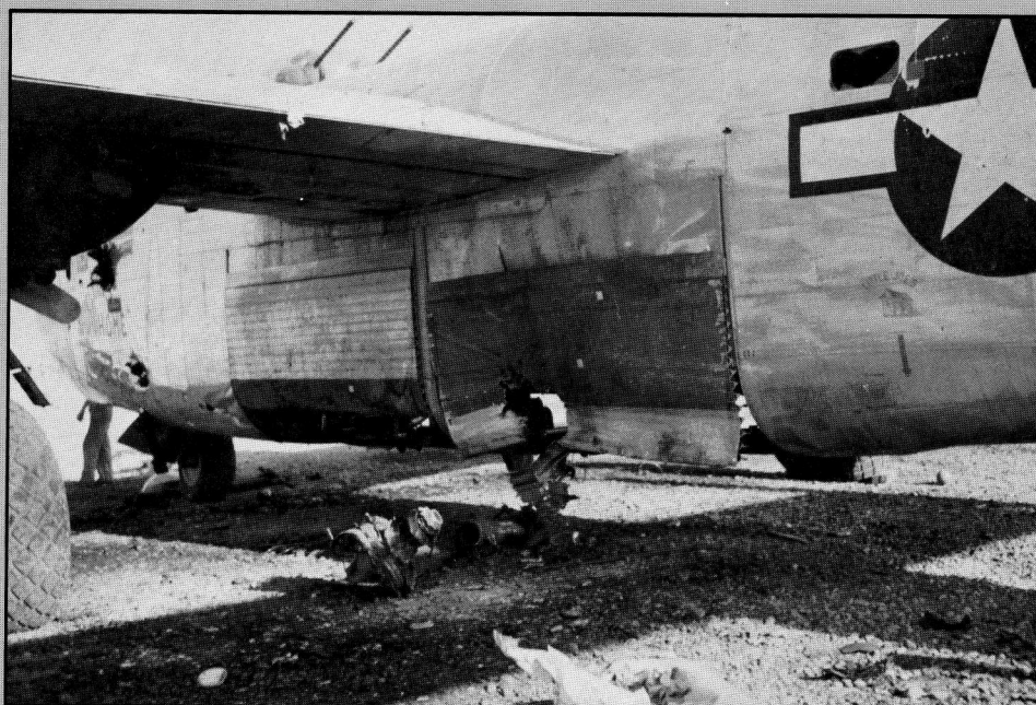
A/C #914 — Damage from explosion 1-9-44.
